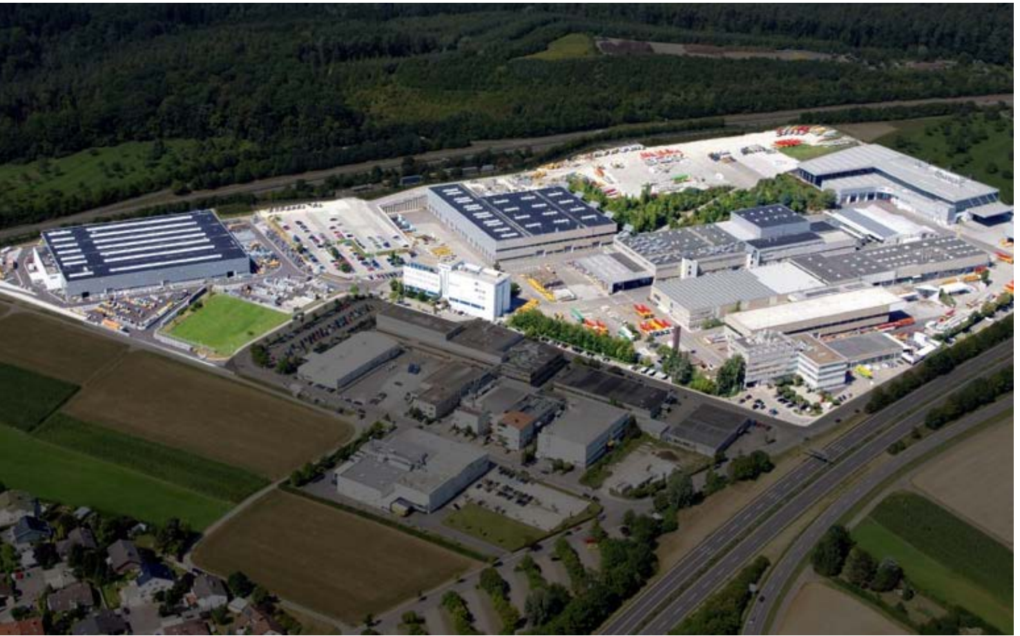
Putzmeister headquarter in Aichtal
