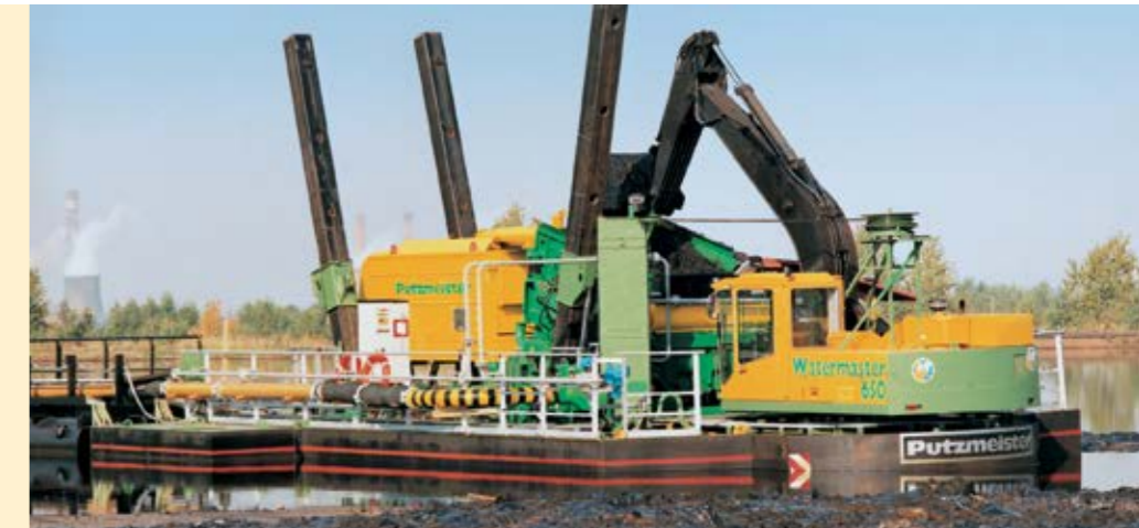
Desludging of a tar dump using a remote-controlled Dredgemaster dredge vessel
