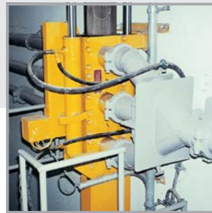
Gate valves for there different delivery lines
