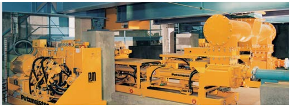
Two KOS 1030 with HA 22 for feeding sewage sludge into the refuse incinerator (Dinan, France)
