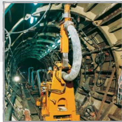
Tunnel concreting with flexible SK pipelines as expansion pipes
