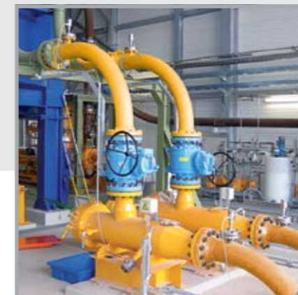
Left: Retained foreign bodies Right: Foreign body separator in a power plant
