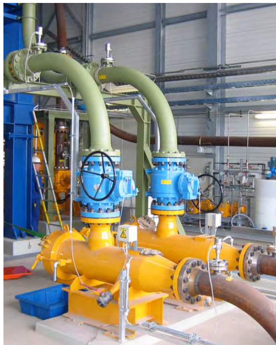
Fig. 114: Foreign body separator on level zero
