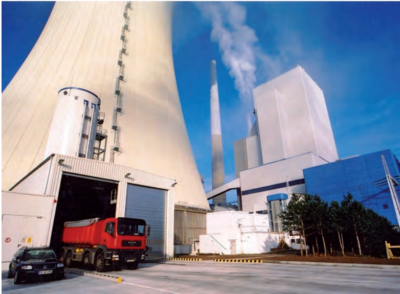
Fig. 111: Sewage sludge receiving station; in the background the storage silo is shown
