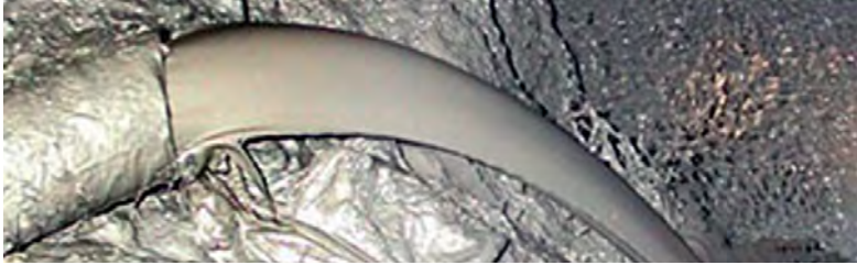
Fig. 149: Backfilling in Lisheen Mine (Ireland)
