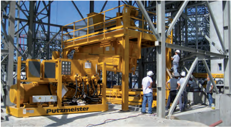
Fig. 81: Zonguldak, Turkey Co-Incineration
