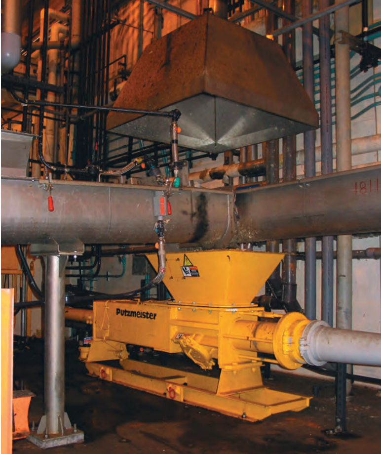
Fig. 29: Single piston pump, type EKO, used in the sewage sludge treatment plant Coney Island New York
