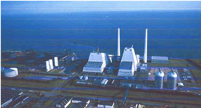
Fig. 45: Avedore power plant Copenhagen
