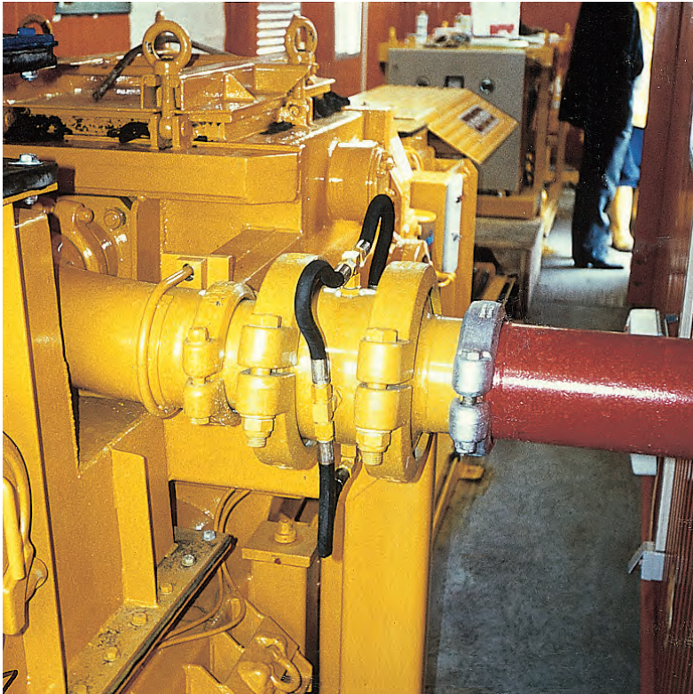
Fig. 131: Injection nozzle directly installed behind the high-density- solids pump
