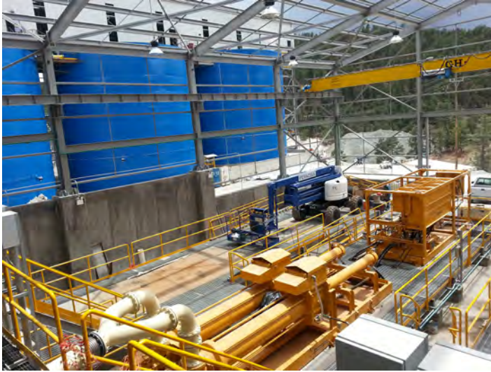
Fig. 142: Installed PCF system with a HSP 25.150 piston pump
