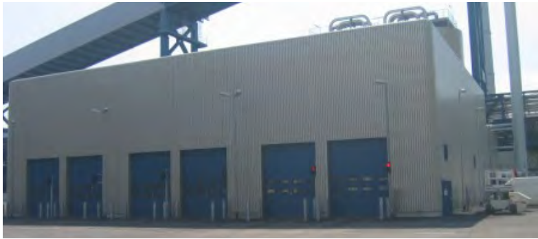
Fig. 37: Sewage sludge receiving hall; In the back- ground the two storage silos, each 850 m 3 capacity
