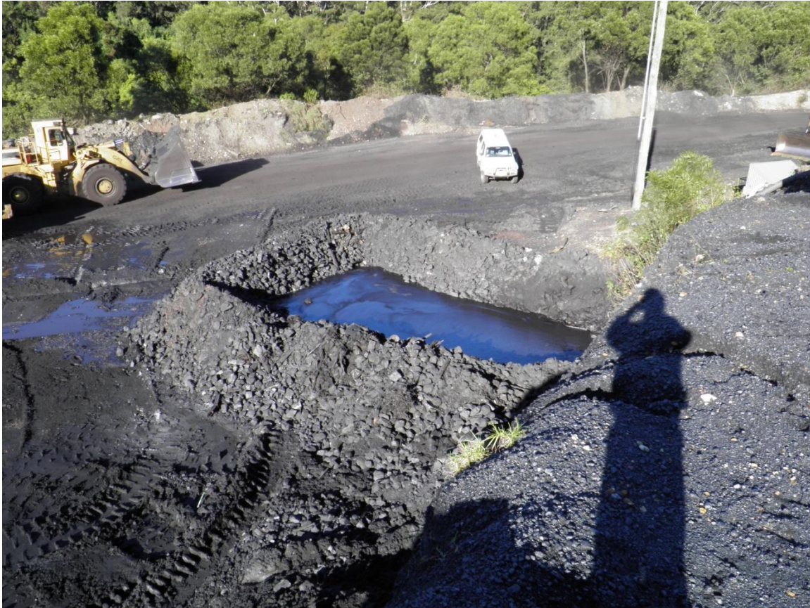
Figure 6: Dam Composed of Loose Rocks
