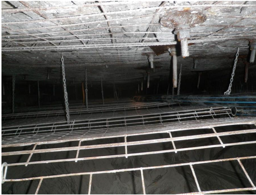
Figure 8: Photo of roof mesh hung to create 'false roof' in PDRR21
