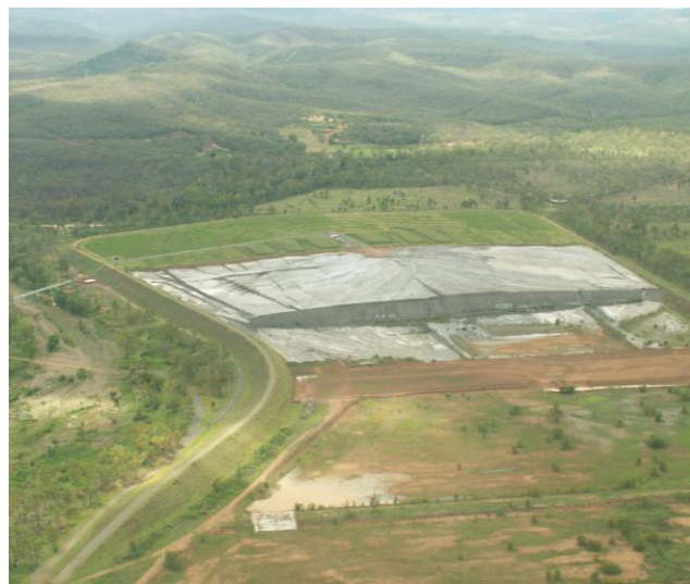
Figure 2 Bund Wall Ash Disposal Site
